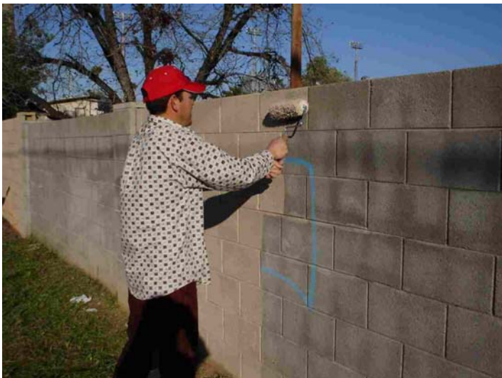
Jose putting the finishing touches!
