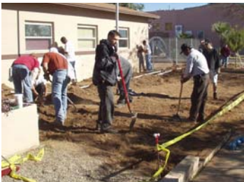
Laying the sprinkler system
